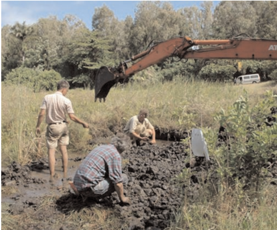
Figure 1. The Dutch team carry out the preliminary excavation.
