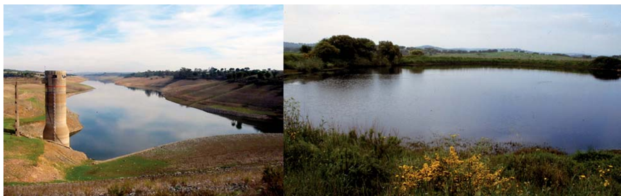
Fig. 3 - Large reservoir (Vale do Gaio dam) – left; small reservoir (Serra de Monfurado area) – right (both in South Portugal) (photos: Nuno M. Pedroso).
