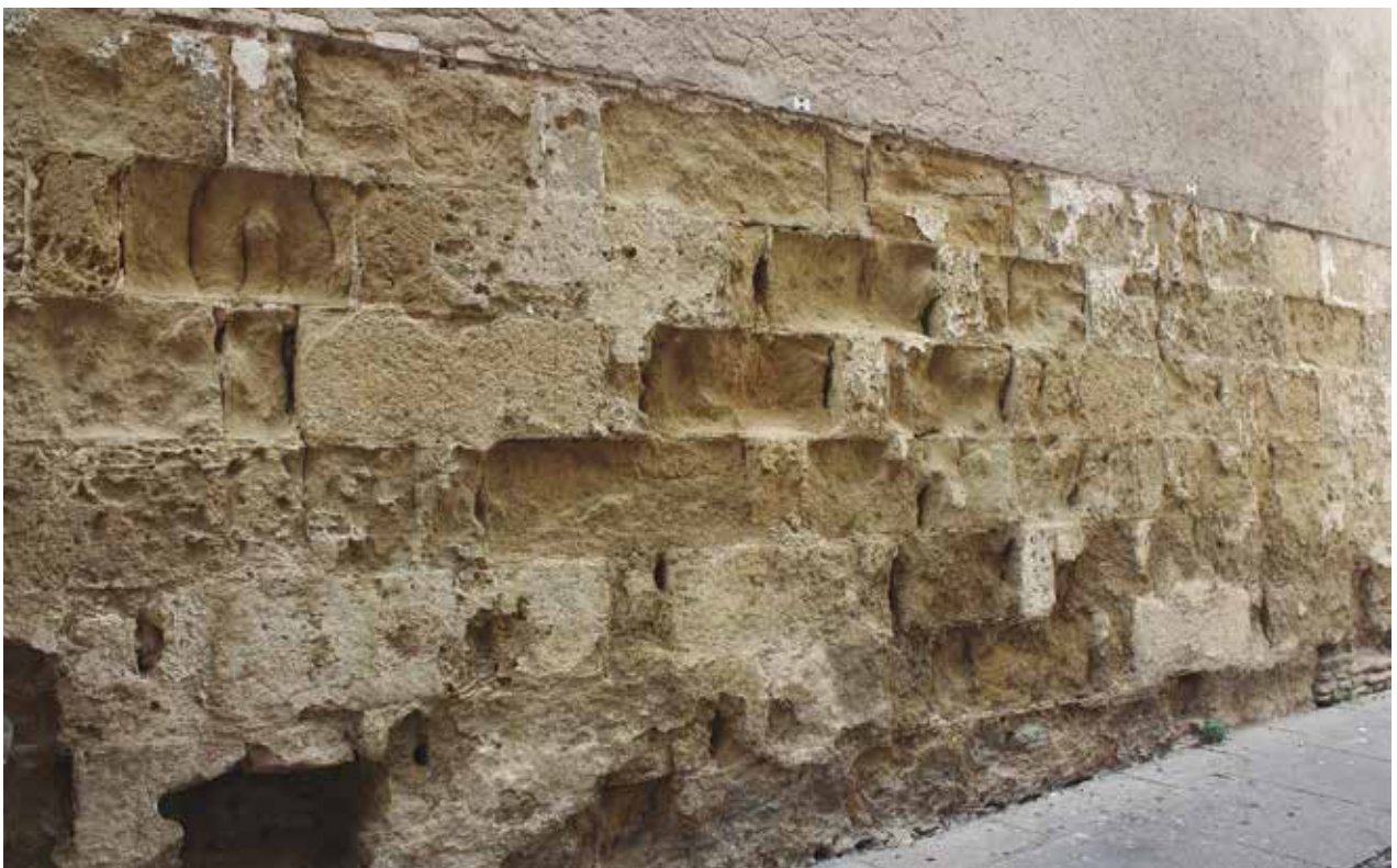
Fig. 12. Córdoba (antigua iglesia de Santa Catalina): vista exterior de las hiladas inferiores que conforman el muro noroeste de la antigua mezquita, en la calle Osio (C. González). / Córdoba (former church of Santa Catalina): external view of the lower line of ashlar belonging to the north-west wall of the former mosque, in Osio street (C. González).
