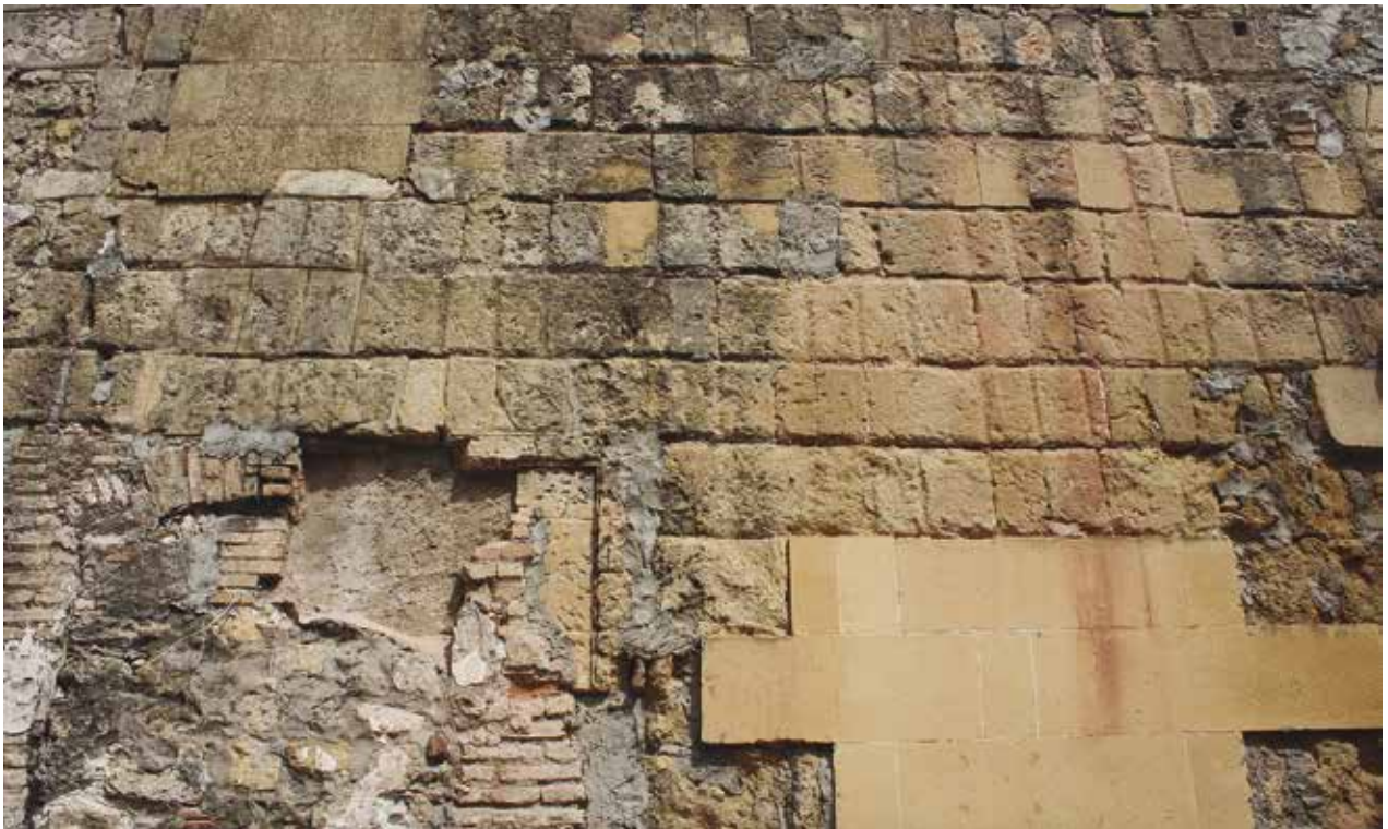
Fig. 11. Córdoba (antigua iglesia de Santa Catalina): vista exterior del muro suroeste en su tramo correspondiente al patio de la mezquita, donde se distingue la labra almohadillada de los sillares (C. González). / Córdoba (former church of Santa Catalina): external view of the southwestern wall, in its section belonging to the mosque's courtyard. It can be observed the padded cut in the stone blocks (C. González).
